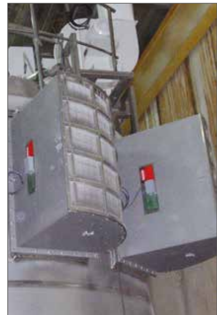
Q-Box II safeguarding a filter housing
