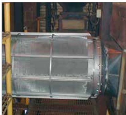
Q-Rohr for protection of a cocoa roasting plant
