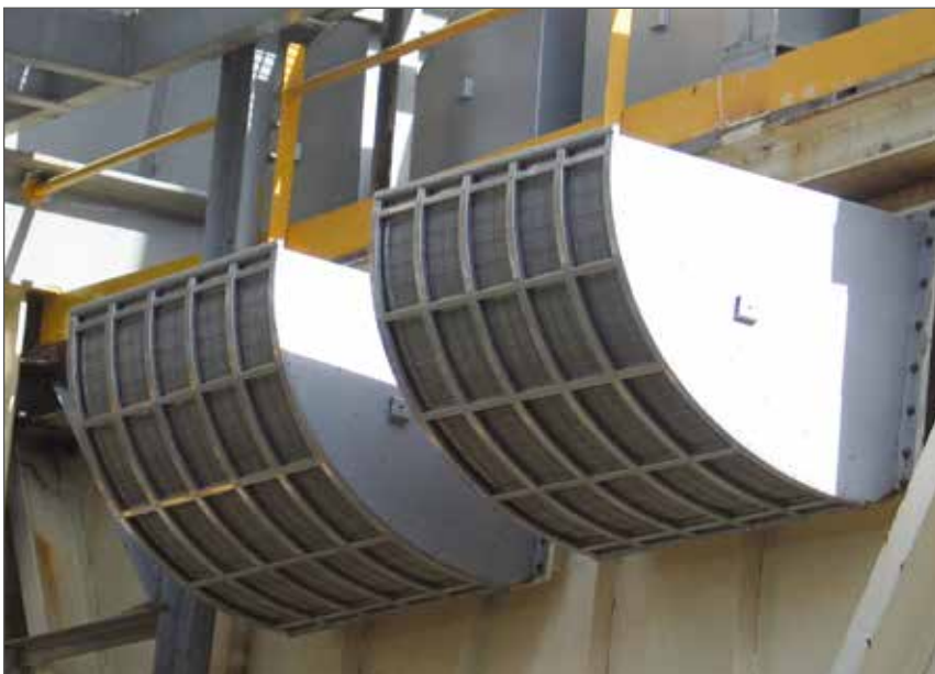
Explosion venting of a wood chip hopper in production of chipboards with Q-Box II: cost-saving production of plant facilities
