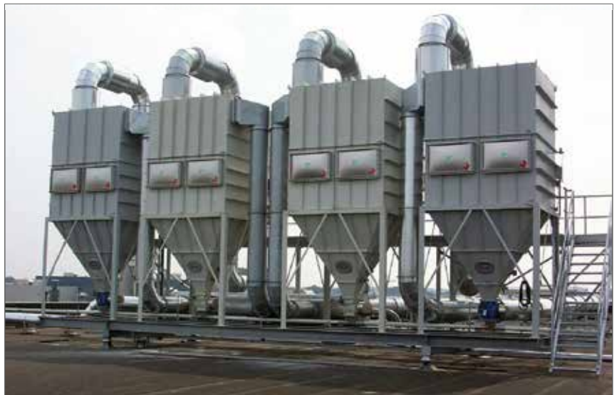
Explosion venting of a filter with EDP explosion panels
